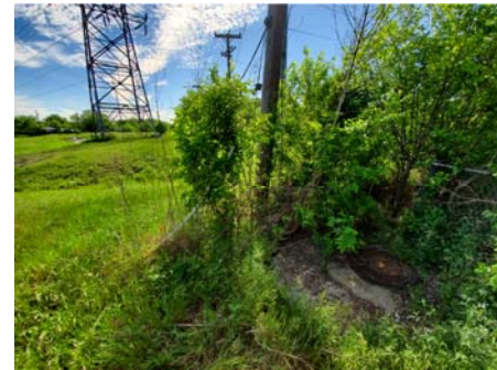
CPS Power Pole Bracing
