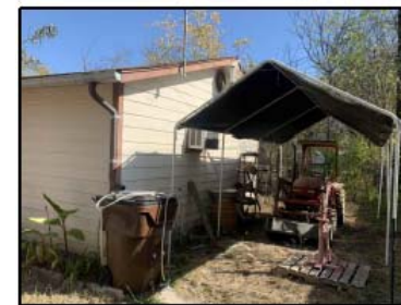
PHOTO #1 SHED LOCATED ON 7826 BRONCO LN.
